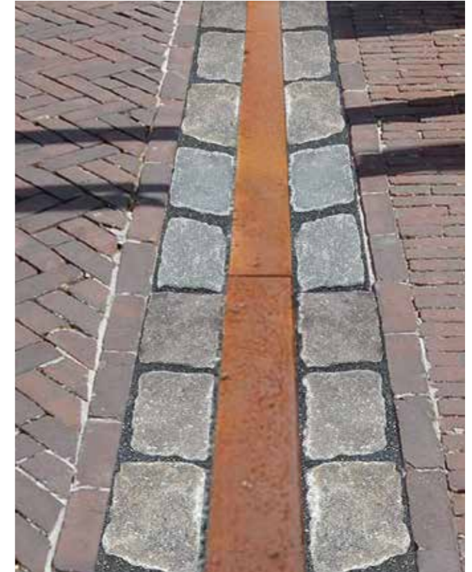
Cortenstalen details in bestrating
